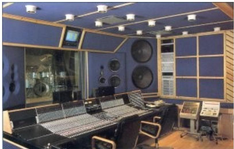
The blue material around the console area is covering absorbers while the back of the room is covered in Scandinavian pine and is therefore reflective
